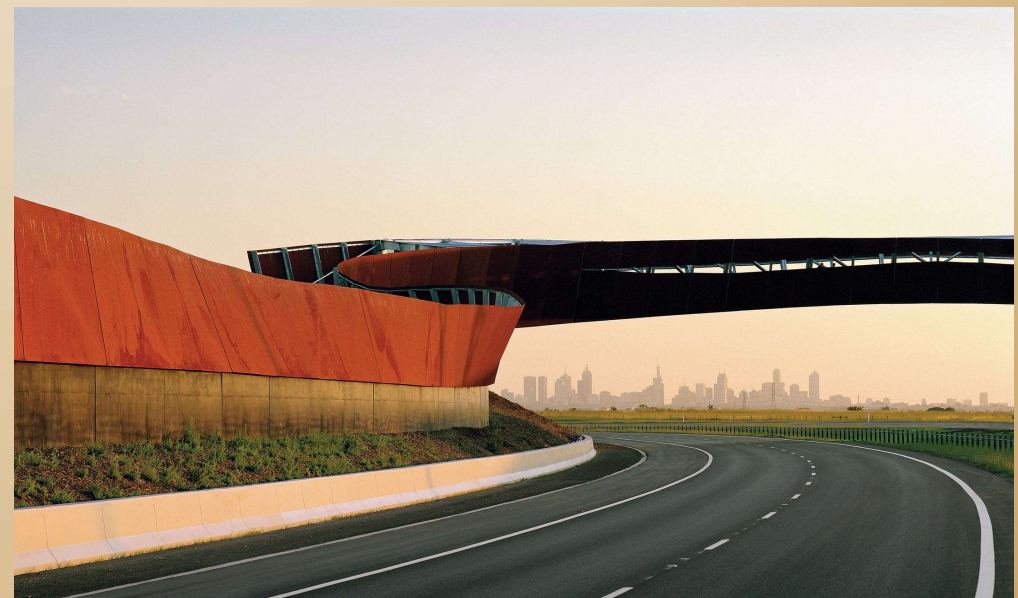
Installation of pedestrian bridge steel and Corten panels
