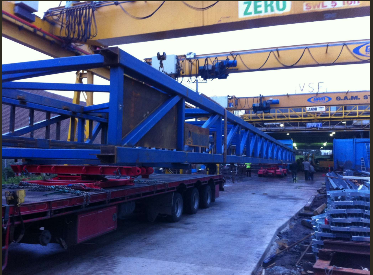
4.5m wide x 45m Long Gantries
